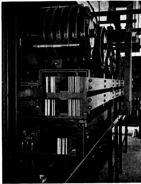
Fig. 6—Generator end of control switchboard, as provided five years ago, rear view. Six 1,000- and 1,500-ampere generators, bus bars terminated for growth when additional units required.
