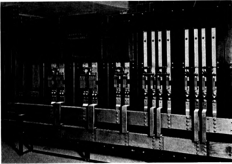
Fig. 1—Incoming direct-current power for large telephone building. About 1,000 h.p. of this is provided to drive motor-generators for reserve central office use, the regular power being alternating current. Both direct- and alternating-current services are duplicated. This panel provides four feeders direct to substation and four to network, capacity 3,480 kw.
