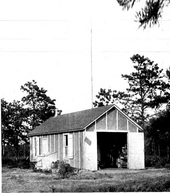
Fig. 5—Receiving test station near Riverhead, L. I. showing vertical antenna projecting through roof of building
