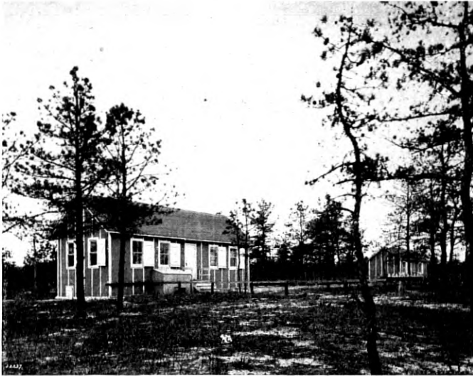
Fig. 2—Exterior of Riverhead Radio Receiving Station
