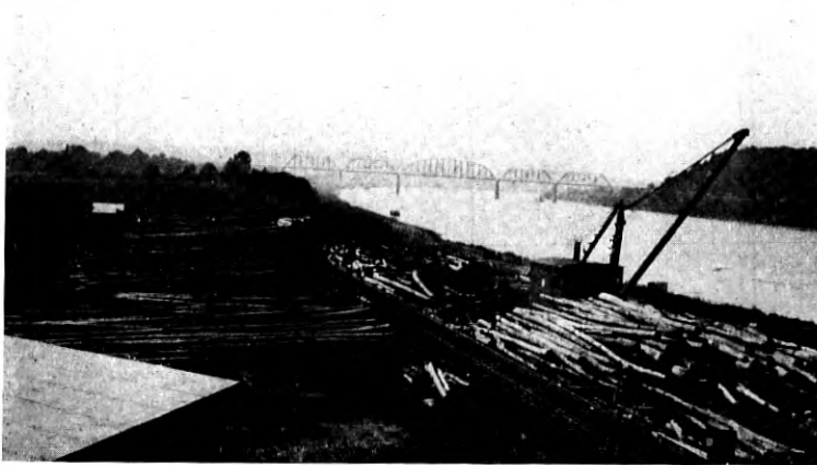
Fig. 12—Derrick for Handling Poles from River Rafts to Piles or Pole Cars in the Yard
