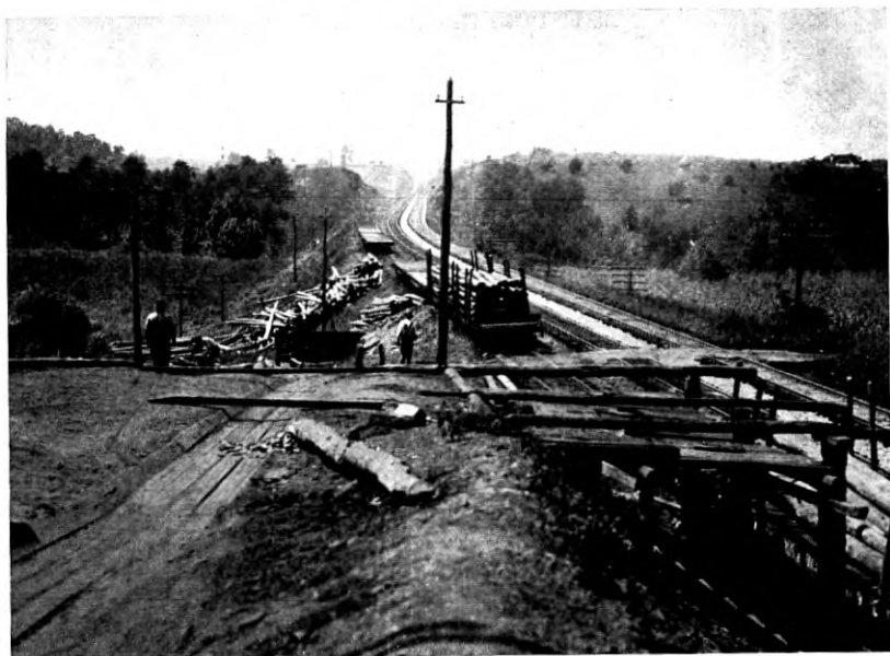
Fig. 9—Unloading Poles at the Shipman Yard
