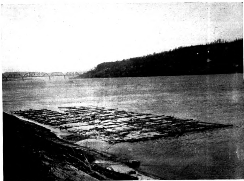
Fig. 10—Four Rafts of Poles at Ceredo Plant
