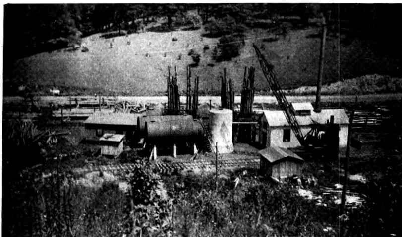
Fig. 22—View of Treating Equipment at Sylva Plant
