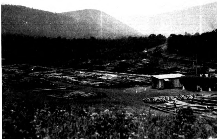
Fig. 2—Portion of Pole Yard at One of the Smaller Plants. (Tool House and Creosote Storage Tank at Right)
