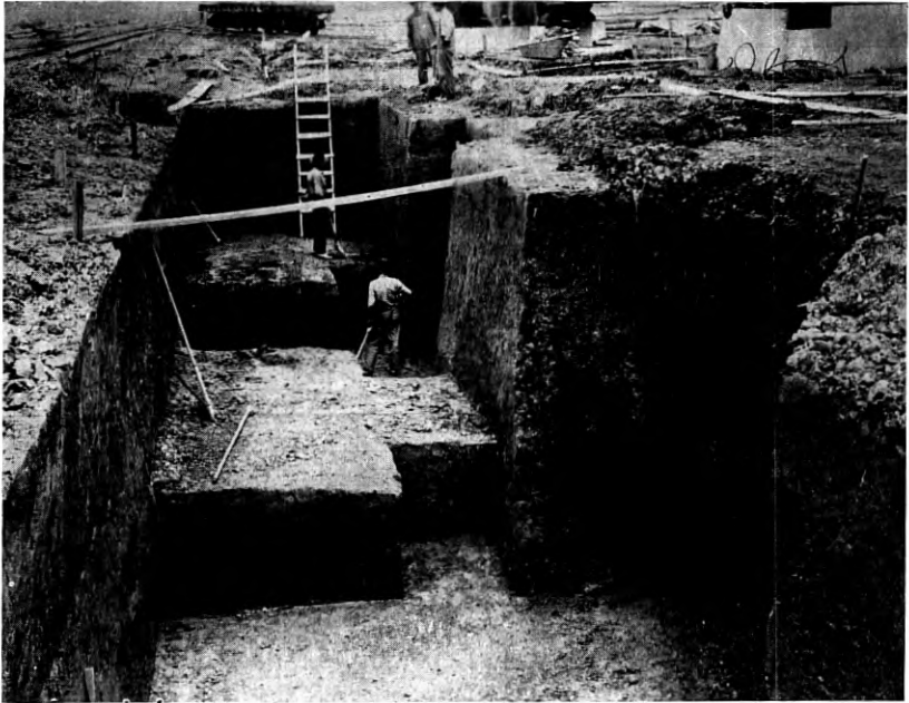
Fig. 24—Excavation for Treating Tanks
