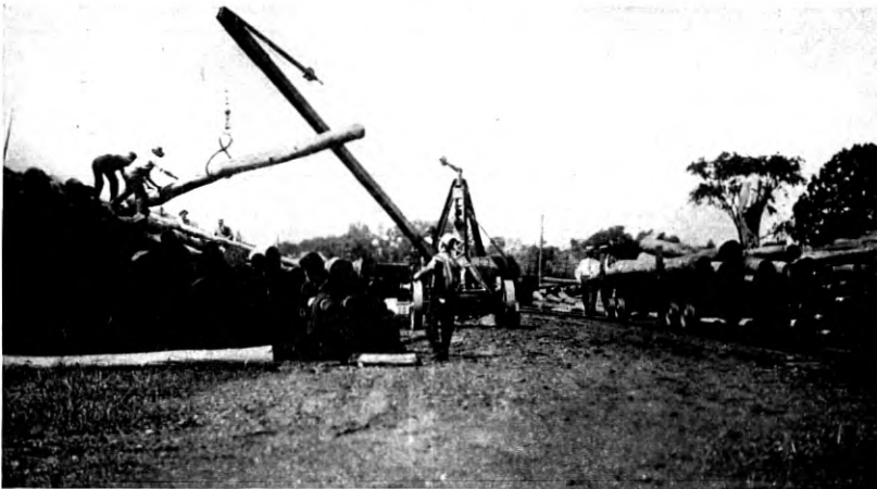
Fig. 14—Tractor Crane Handling Poles from Rail Dollies in Danbury Yard
