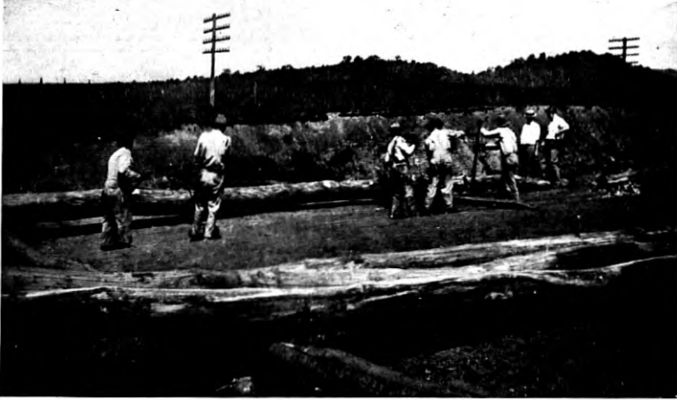
Fig. 13—Handling Poles by Man Power
