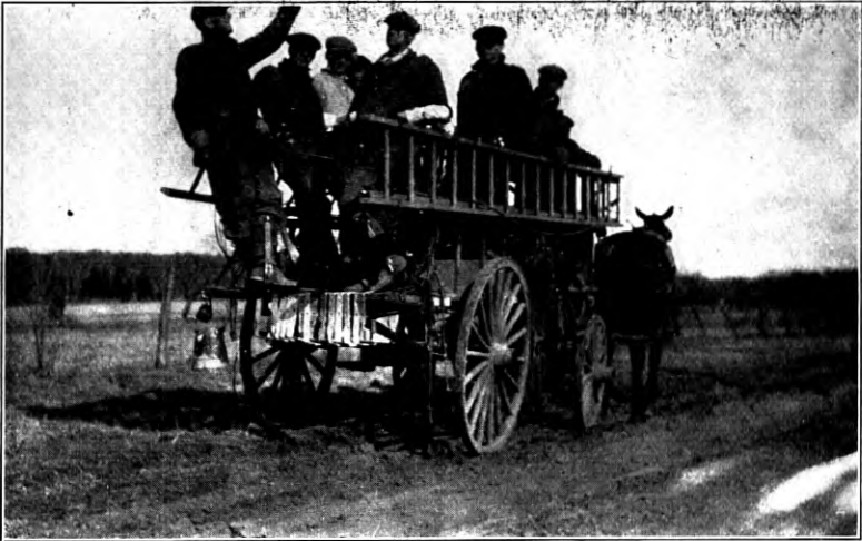
Fig. 3—Heavy Construction Truck Carrying Gang, Tools and Materials, 1896
