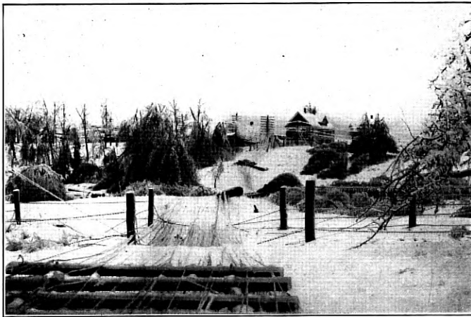
Fig. 3—Damage to Section of New York-Boston Main Line Near Worcester, Mass. Storm of November 28, 1921
