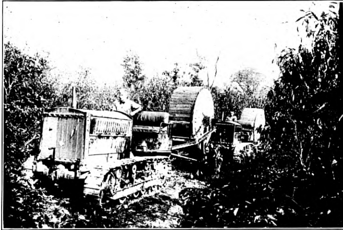
Fig. 12—Tractors Placing Cable Reels in Rough Country
