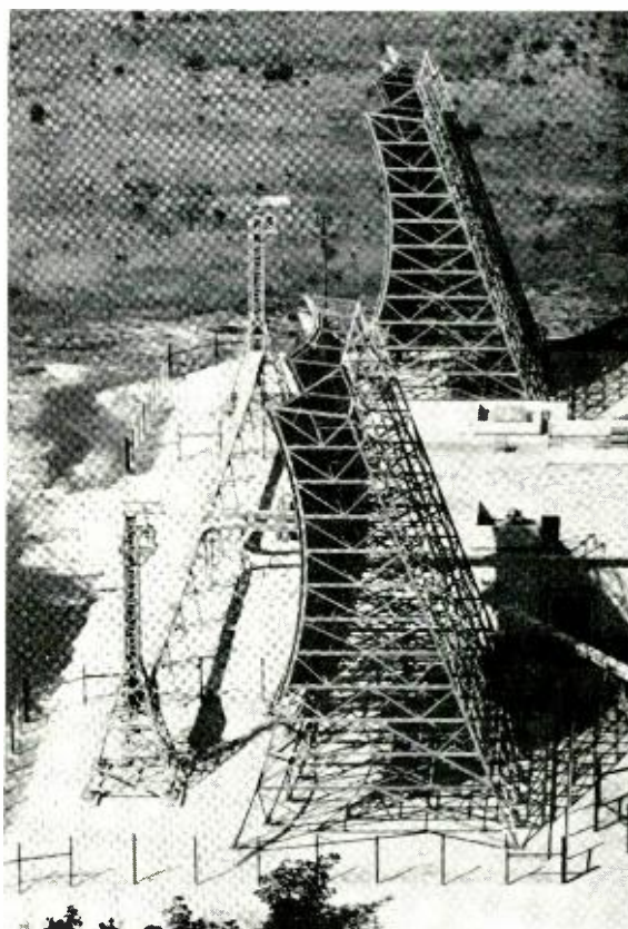
Over-the-horizon antennas located at Florida City, Florida, link the United States with Cuba.
