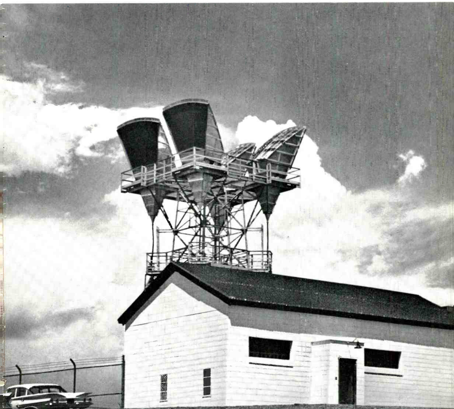
TH Tower at Rawlins, Wyoming
