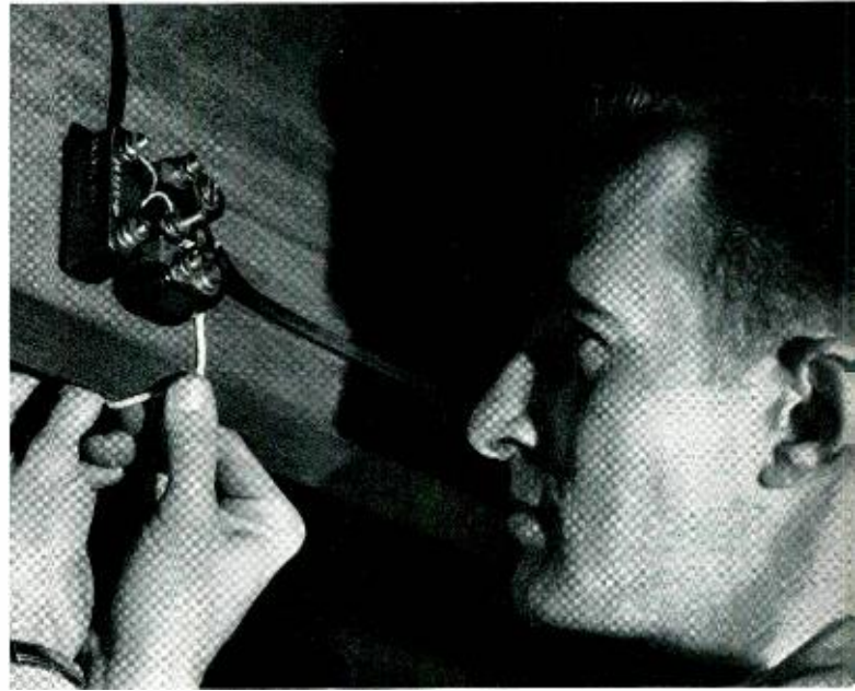
The author examines a station apparatus protector which has been mounted on premises of a customer for his and the telephone's protection.
