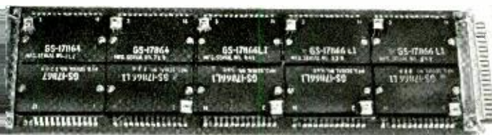
Fig. 3 — An example of printed wiring used to interconnect several sub-modules on a single board as used in a transistorized high-speed digital computer circuit.
