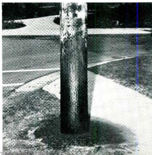
Fig. 1—When the critical retention is exceeded, a pole may "bleed" some of its preservative.
