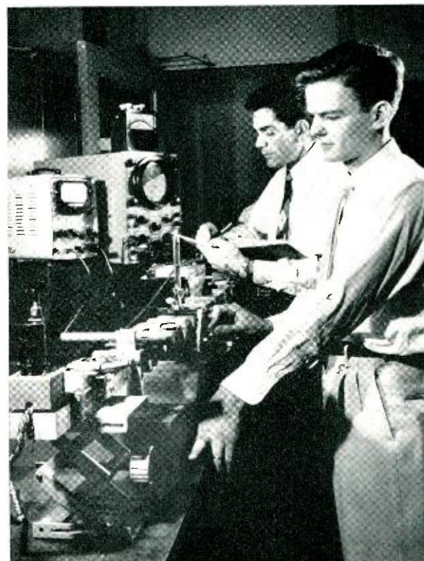
J. J. Kostelnick and F. J. Sansalone testing field-displacement ferrite isolator.
