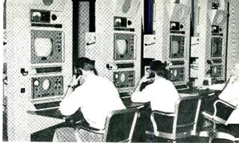
Television operating center in Chicago. Standard operating center equipment was designed to coordinate program elements and monitor video quality for both incoming and outgoing television transmission.
