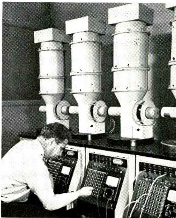
Fig. 2 — The author makes a further electrical check of a relay contact that has registered "open".
