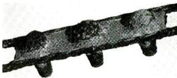
Fig. 7 — Cable clamp showing extreme corrosion from exposure to industrial atmosphere.
