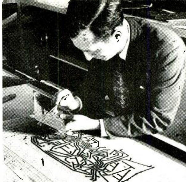
Fig. 4 — A Western Electric draftsman uses black tape to lay out a circuit to agree with an engineering model of a printed-circuit board.
