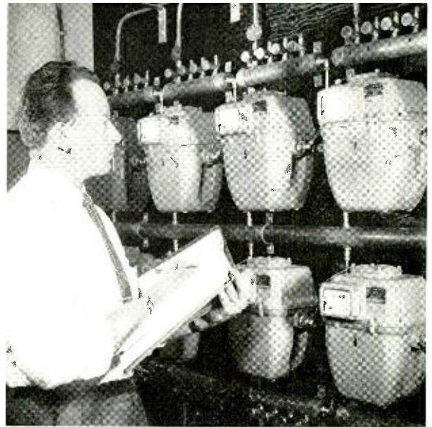
Fig. 2 — G. W. Hausold, New Jersey Bell switchman, records dry air flow to exchange cable systems.
