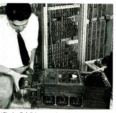
Fig. 2 — T. J. Palermo attaching photographic film holder to oscillograph; six mirrors for reflecting light to the film are in compartment at right.
