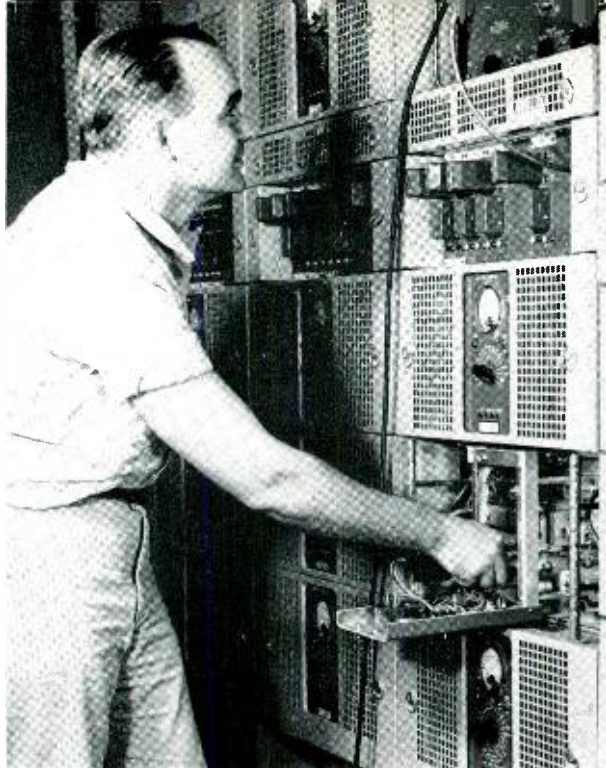
Fig. 5 — Donald H. Depew of the Long Lines Department of A.T.&T. adjusts an initiator while watching the test meter.
