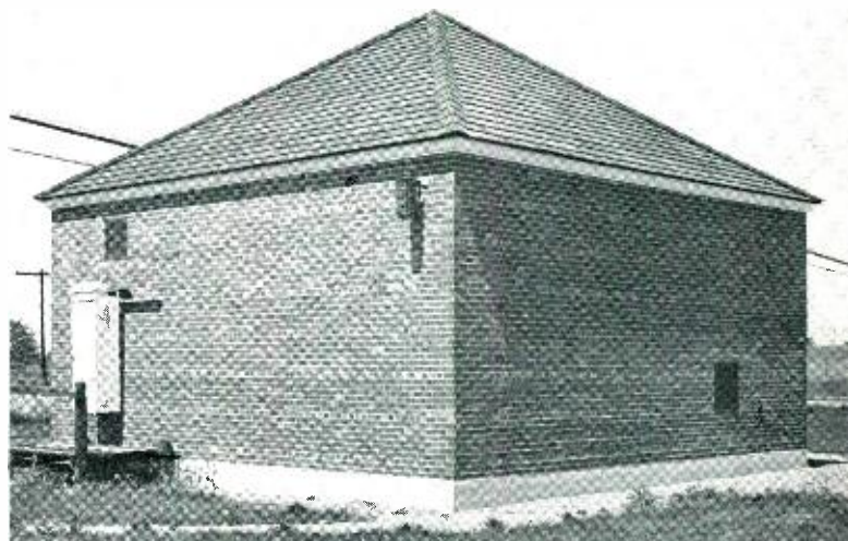
Fig. 5 — An N repeater cabinet mounted on the outside of an unattended K repeater station.
