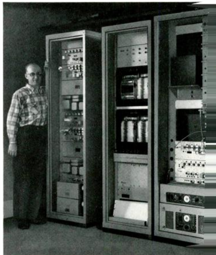
Fig. 6—Some of the receiving and recording equipment used in the year-long over-the-horizon tests.
