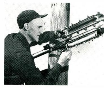
Fig. 2 — T. E. Edwards, now returned to the New Jersey Bell Telephone Company, installing a mechanical splice case at the Chester Laboratories. This case was subsequently tested in a general field trial and has become standard
