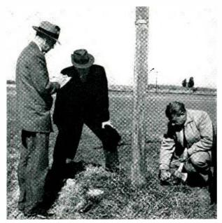
Fig. 5—Engineering inspection of a field trial pole; left to right, J. G. Sullivan, New Jersey Bell Telephone Co., E. Weller, A.T.&T., and A. H. Hearn, Bell Telephone Laboratories. Mr. Hearn is prodding ground line section of pole prior to taking core sample to determine internal condition.
