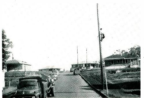
Fig. 1—Installing field trial sec tion of new urban wire new Atlanta, Ga. Sites were chose to test the wire under variou distribution conditions, inclue ing service to new housing de velopment shown here.
