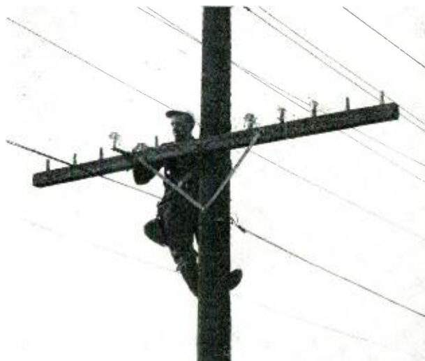
Fig. 4—W. R. Kelly of the New York Telephone Company checks the wires on a tandem bracket. This is a point-type bracket with only two insulators, used on voice-frequency lines; a double-skirted insulator at the right takes the place of a drop bracket.
