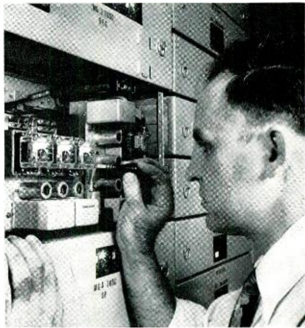
Fig. 2—A. J. Uminowicz adjusting meters in an L3 terminal amplifier at the Laboratories. One such meter in each electron tube circuit is adjusted to read 1.0 arbitrary units of plate current when a new tube is inserted. As the tube loses emission with age and the current drops below 0.65 of its original value, a contact on the meter pointer closes, actuating an alarm that indicates the end of the useful life of the tube. This feature supplants the routine periodic tube tests required in other circuits to prevent total failures that would interrupt service.
