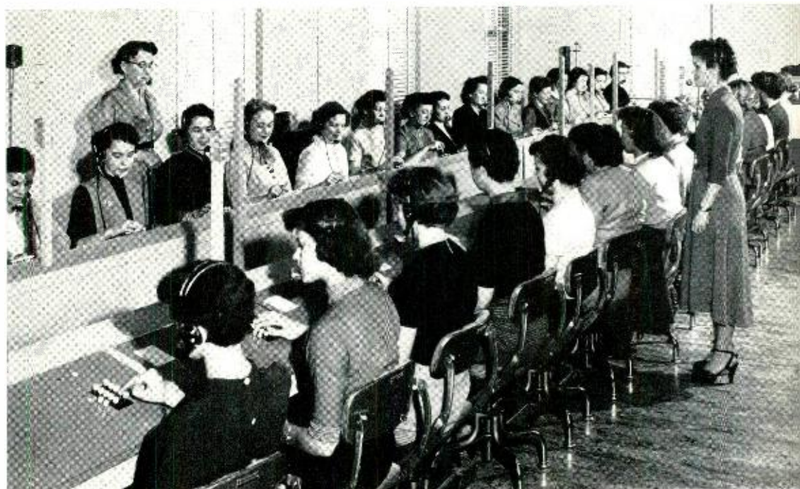
Operators at recently installed switchboard, Uptown Toll Center, Washington, D. C.
