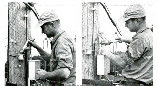
cable, heating asphalt and handling hot material, and making constrictions in the sheath. Tools and materials for the resin method are light in weight, compact, and can be carried up the pole in pouches attached to the body belt of an individual workman.
