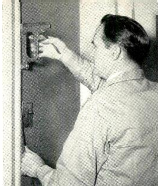
Installer D. Keegan of the New York Telephone Company staples JKT wire to run inconspicuously along doorway trim.
