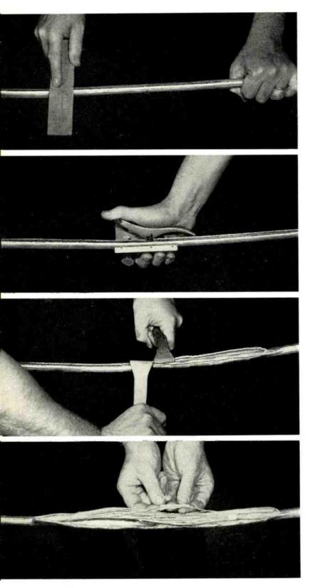
Cleaning lead sheath preparatory to use of the cable sheath slitter is essential to the final soldering operation.
