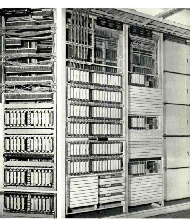
Fig. 7 (left)-A district group connector frame, which is required only in No. 1 crossbar offices. Fig. 8 (right)-A transverter connector bay at the left, a calling line register bay in the middle, and a bay of senders at the right in the Hackensuck office.
