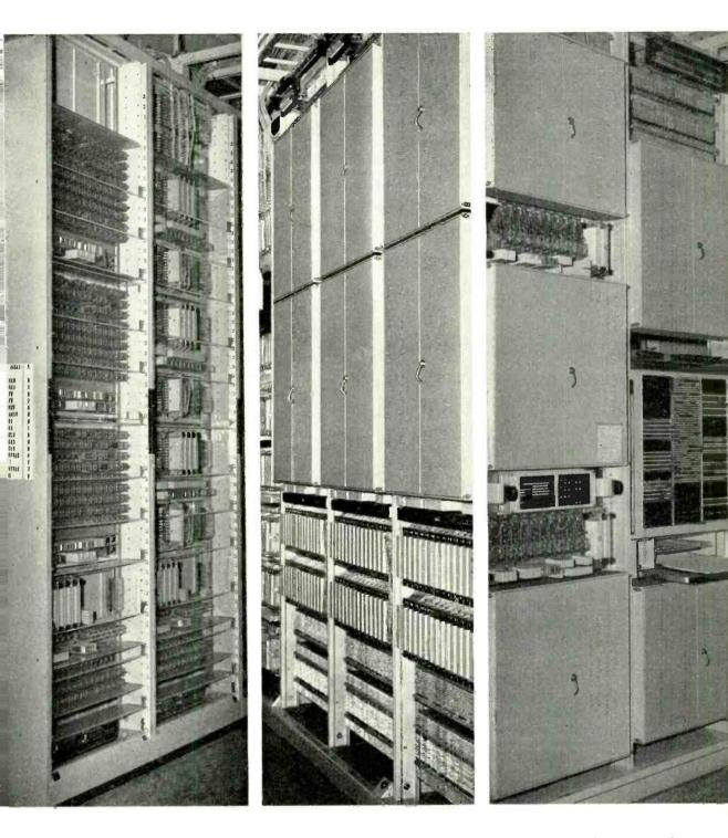
Fig. 3 (left)—A recorder frame in a No. 5 crossbar office in Englewood, N. J. Three recorders occupy the upper three quarters of both bays of the frame, while two call identity indexers are at the bottom of the frame—one call identity indexer in each bay. Fig. 4(center)—Three transverter frames in the No. 1 crossbar office at Hackensack, N. J. Fig. 5 (right)—The master timer frame at the left and the transverter trouble indicator frame on the right in the No. 1 crossbar office at Hackensack.
