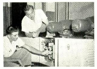
Fig. 5–The two motor alternator sets with the dc motor starters and motor controls.
