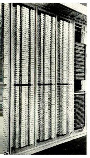
Fig. 3-A bank of E1 repeaters installed in the central office in Jamaica, Long Island.
