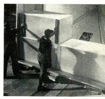
Fig. 6–Placing the lens section in the housing.
