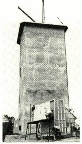
Fig. 7-A lens being assembled on the ground preparatory to hoisting to tip of tower.
