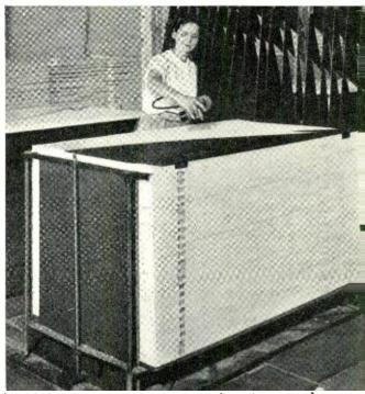
Fig. 2—After an aluminum template is properly placed it is sprayed around the edge to mark its position on the slab.
