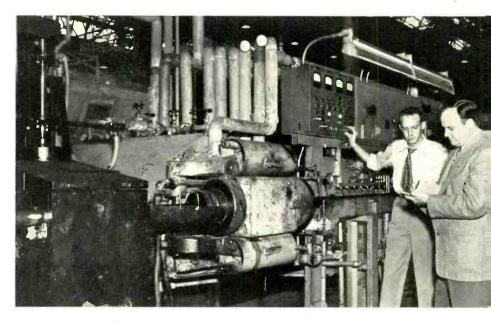
C. R. Noble (right) with E. D. Long (Western Electric) review the operation of the plastics extrusion machine for applying the polyethylene jacket to a Lepeth sheathed cable core. The cable core enters the extrusion die at the left, and the covered core emerges from the die to enter the water trough just below Mr. Long's right arm.
