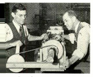
Above, R. B. Ramsey (left) adjusts the thermostatic switch in the test set-up for making measurements on a section of K cable under controlled temperature conditions. R. A. Ragan, Western Electric craftsman, is placing a cover on the refrigerant container.
