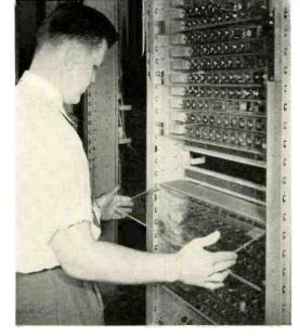
Front view of translator and route relay frame showing method of removing front covers.
