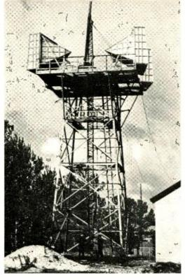
The "golden spike" station of the Bell System's transcontinental radio relay route at Crow Creek, Wyoming.
