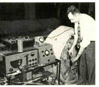
R. A. Kempf is preparing a test arrangement to make measurements on a reel of coaxial cable under varying temperature conditions.
