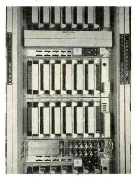
Fig. 4 (above)—On this line link connector frame, the jack strips in the face of the frame uprights are plainly evident.
