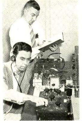
R. L. Wallace (left) balances an AC bridge to measure the impedance of a transistor as W. J. Pietenpol records readings.
