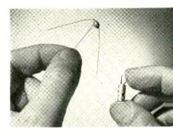
Significant advances in the development of the transistor, a tiny amplifying device which has been called the first serious rival of the vacuum tube, were recently announced by Bell Telephone Laboratories. The transistor was invented here three years ago. Most important of these advances is the construction of operating samples of a radically new type of transistor which has astonishing properties never before achieved in any amplifying device.
