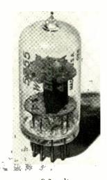
A recent addition to the increasingly popular family of miniature tubes is the Western Electric 5755/420A. This is a doubletriode tube having separate indirectly heated cathodes.
