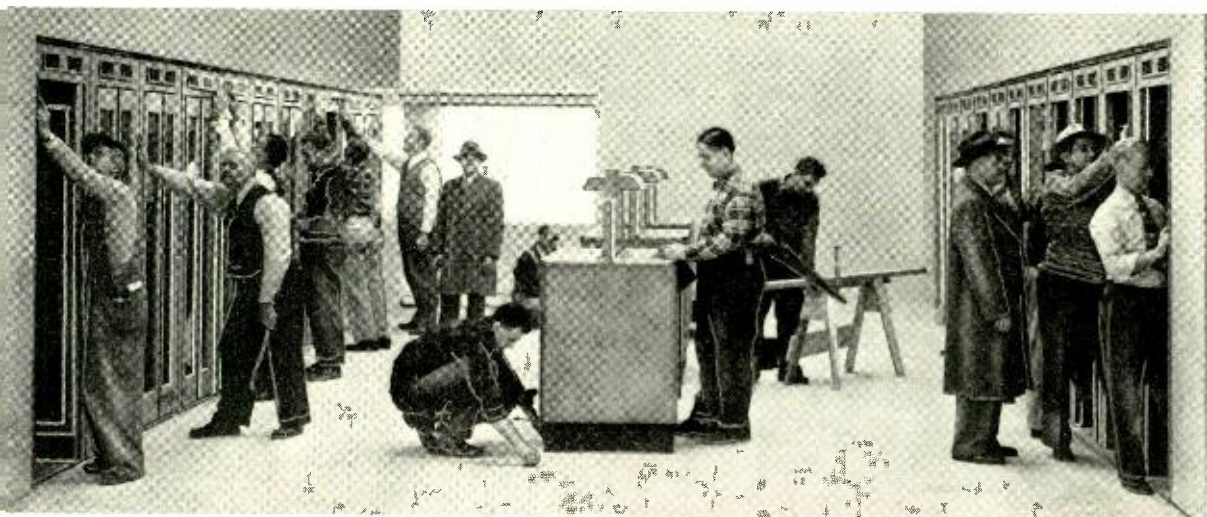
Installing coin telephone booths in the new Port Authority Bus Terminal.
