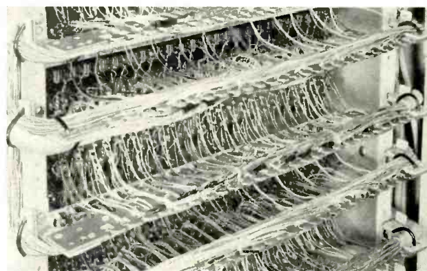
Left—Sewn cable forms at the rear of the four-wire voice frequency bay equipped with 410A jacks. Right—Use of new fanning strips with the 482A jacks provide greater accessibility as well as neater appearance at reduced cost.
