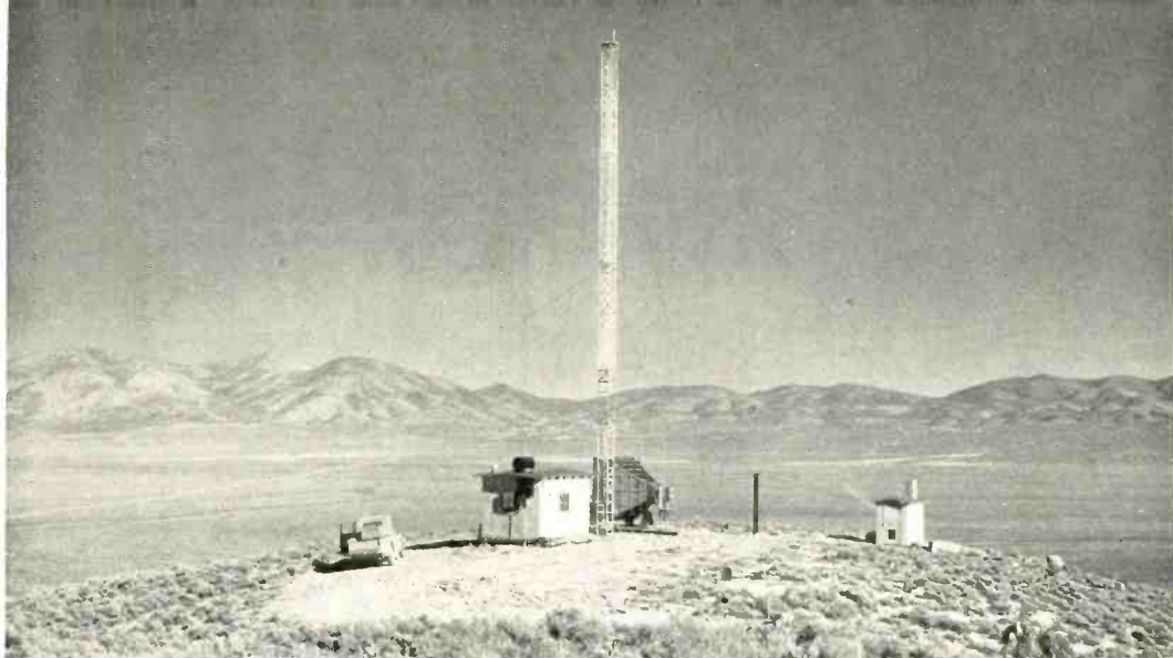
Transmitting station on spur of Table Mountain. The tower is used for loss vs height and the horn for loss vs time measurements.
