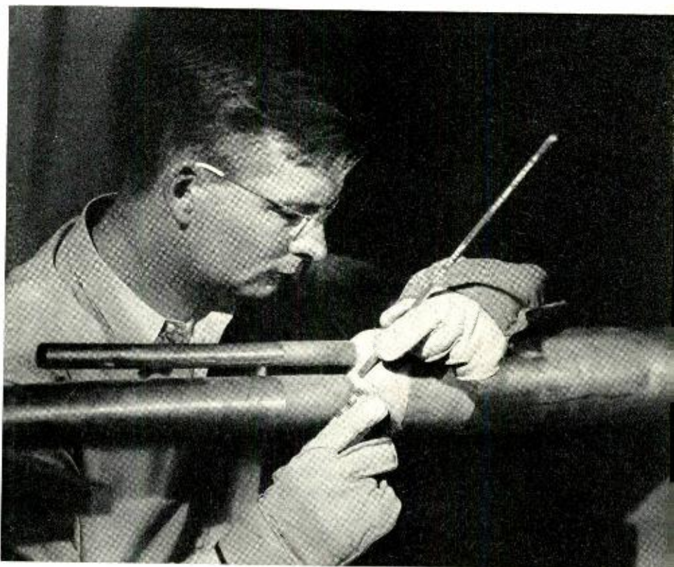
Method of applying sealing solder to a branched joint.
