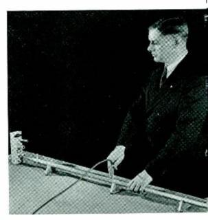
Fig. 1–J. L. Wenger attaches a coaxial lead from a vacuum tube voltmeter to one of the three voltage taps on a 75-ohm coaxial impedance standard
