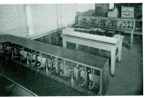
Fig. 4 - A multiple listening position is placed at each side of one of the terminal positions
