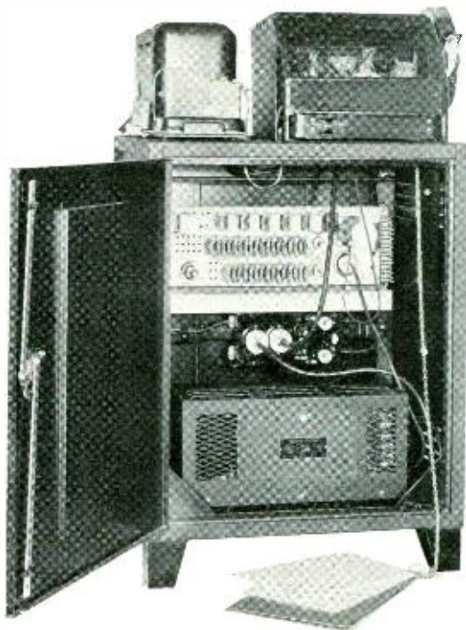
Fig. 3—Navy transmitting equipment for teletypewriter transmission over submarine cable
