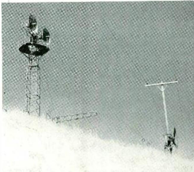
Fig. 3—Antennas as used on Mount Orizaba, Catalina Island, for test over the path to Soledad Mountain. Second receiving antenna attached to pole fifty feet lower than others
