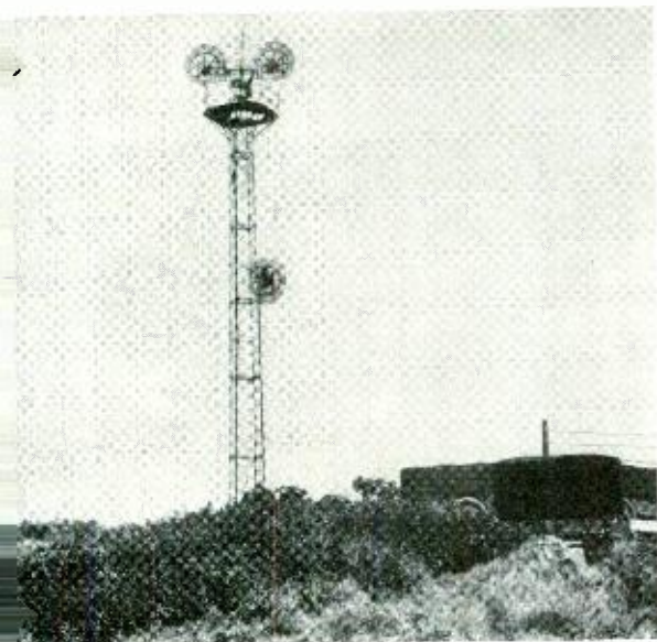
Fig. 2—Antenna site on Soledad Mountain showing a receiving antenna twenty-five feet below the regular set which was used in the studies of complementary space diversity reception
