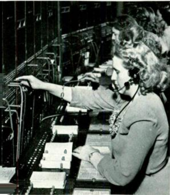
board modified to become a No. 6 toll board
