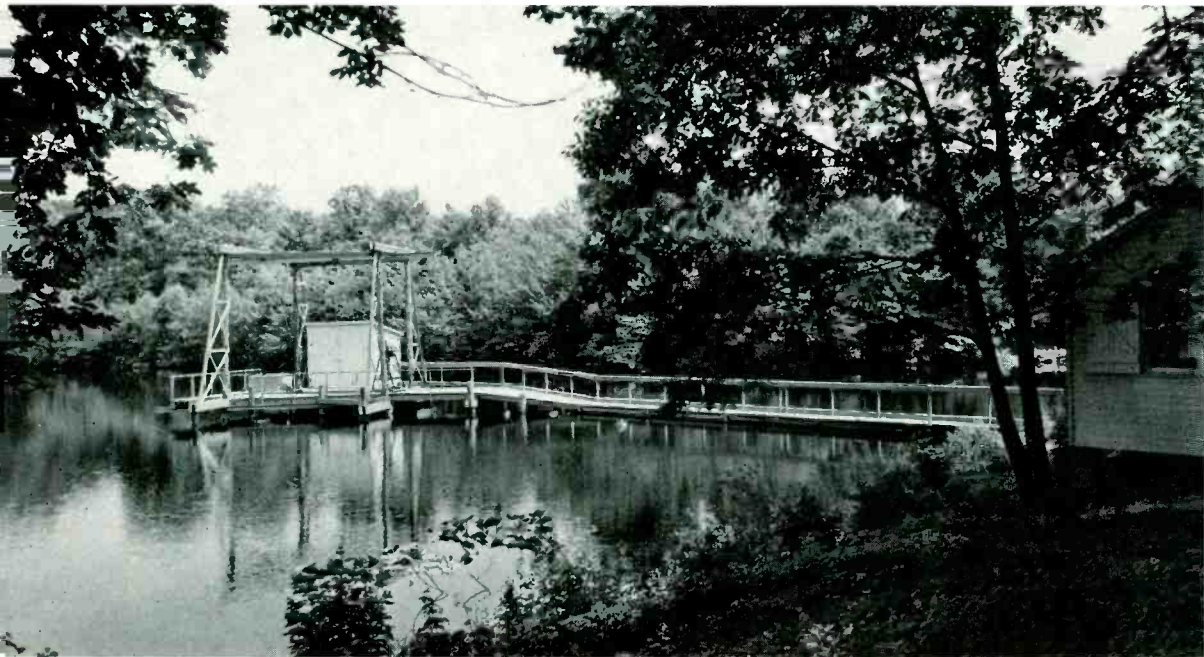
Sonar test station at Birchwood Lake, Mountain Lakes, New Jersey
