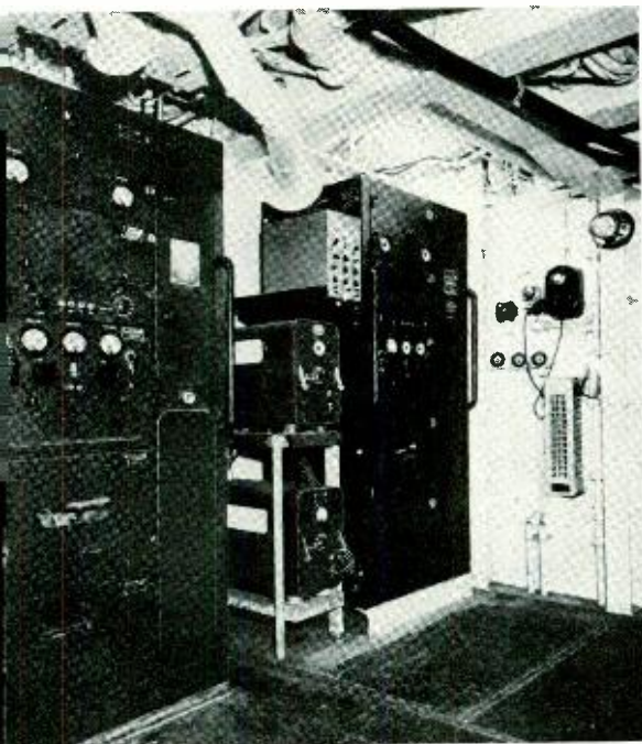
Main frame installation of Mark 3 and Mark 4 radars
