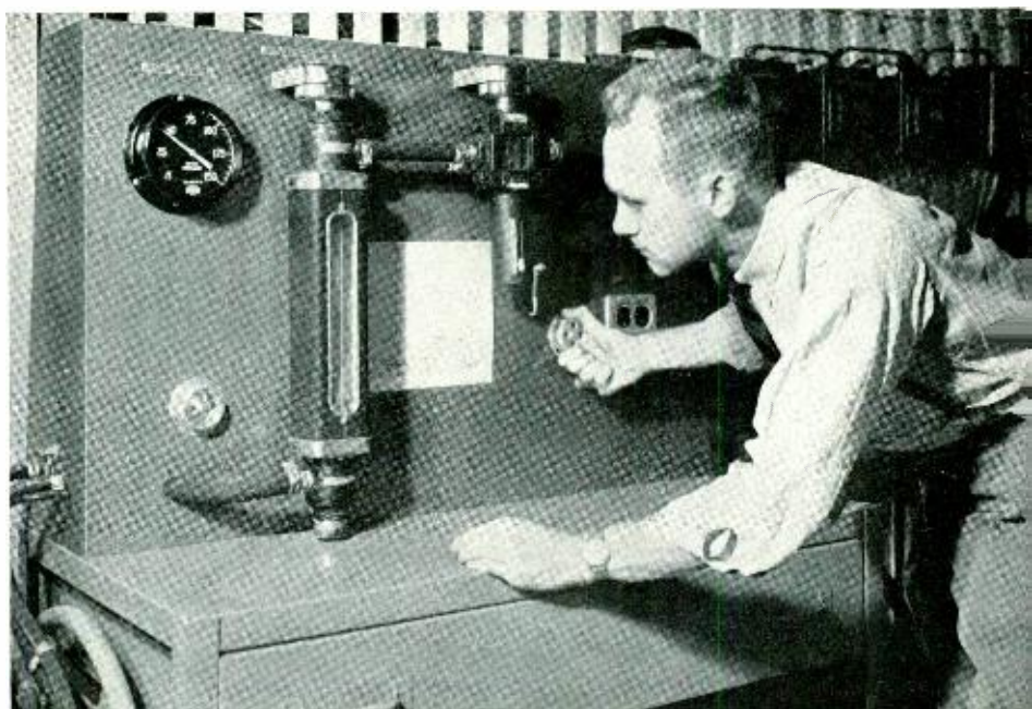
J. Leighton is regulating the water supply for cooling the dummy antenna for the 10-kw broadcast transmitter
