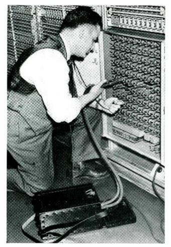
ANY electrical contacts are closed and opened in relays and other switching devices that operate in telephone circuits each time a subscriber calls. The contacts are usually made of precious metal welded onto springs near their outer ends. These metals provide dependable service for a long time, but eventually mechanical abrasion and electrical erosion require that they be replaced.
