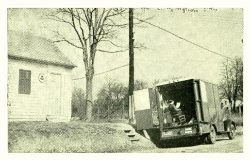
Bell Laboratories test truck making transmission measurements on power-line carrier circuit just outside a rural central office
