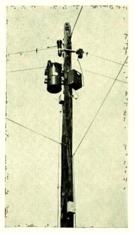
Subscribers would be connected to the power line through a coupling unit consisting of condensers and a transformer installed on a cylindrical core as shown at the left near the top of the pole beneath the power-line lightning arrestors
