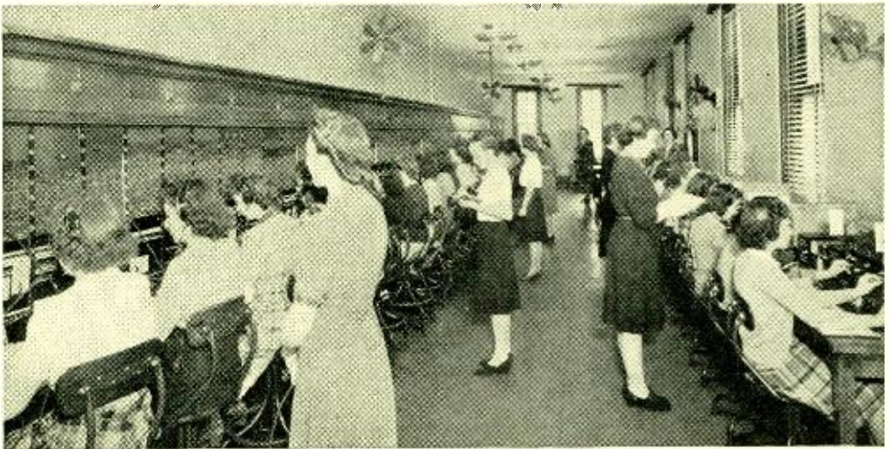
New supplementary toll positions in the Vincennes, Ind., operating room that went into service about October 1. Toll board at left and supplementary positions at right. These positions are described by B. C. Bellows on page 110 of this issue
