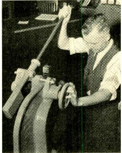
H. E. Pearsall punching holes for mounting vacuum tube sockets on a metal chassis in the Transmission Development Laboratory Shop
