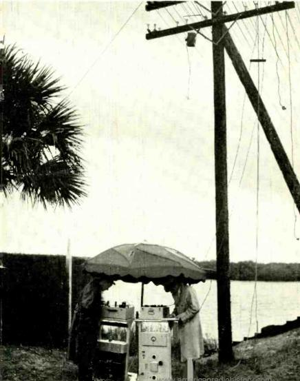
A 1500-foot cable crossing of the Loxahatchee River, on the Charlotte-West Palm Beach system, presented unusual loading problems. The cable is the four-wire discinsulated type. Loading is being adjusted and the cable is being balanced, in this photograph by W. H. Tidd.
