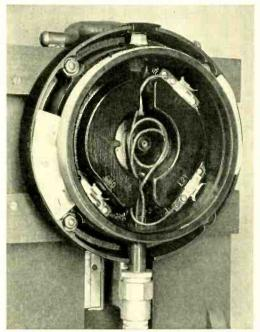
Fig. 1—The base of the new set provides termination for the wires and is designed to support the housing and to mount on a wall, either directly or by use of a backboard October 1940
