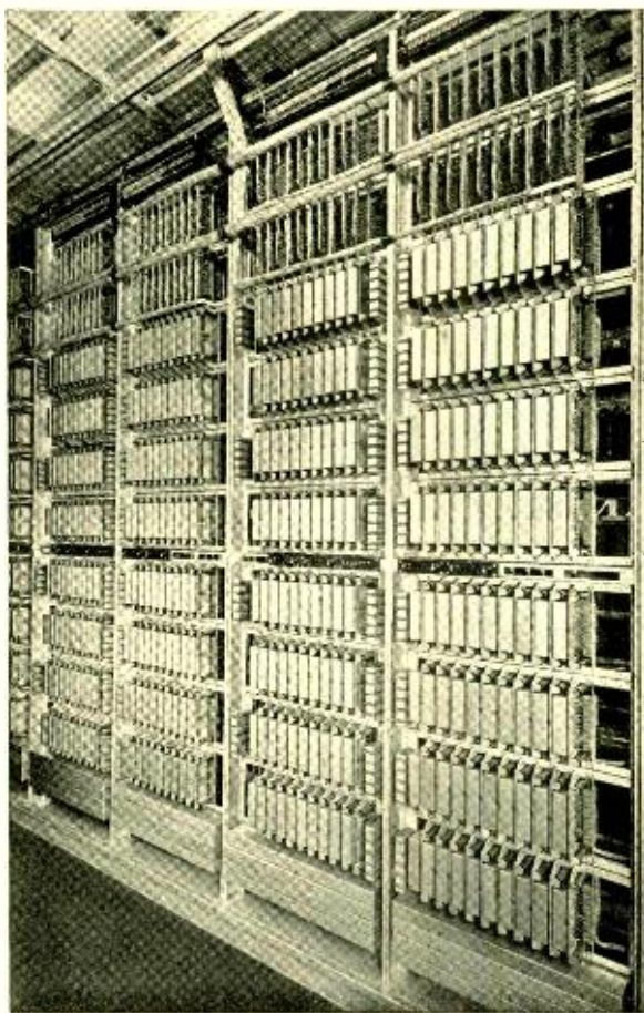
Fig. 1—Number-group connector frames in the Murray Hill-6 Office on East Thirtieth Street
