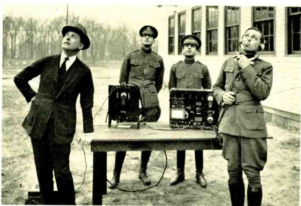
E. B. Craft, Ralph Bown, Nathan Levinson and N. H. Slaughter using early Western Electric apparatus to carry on two-way conversation with an airplane
