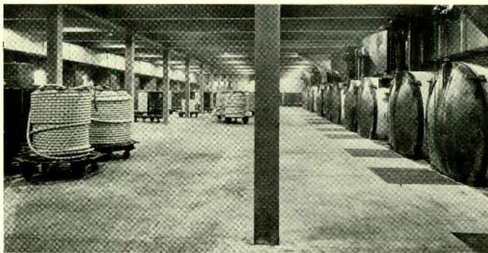
The storage room at Point Breeze showing the ends of the vacuum tanks used for unloading
