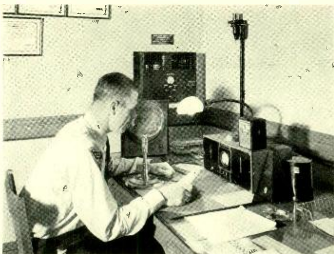
Fig. 5—On the wall in front of the dispatcher is a time signal device and on the desk in front of him is the speech amplifier
