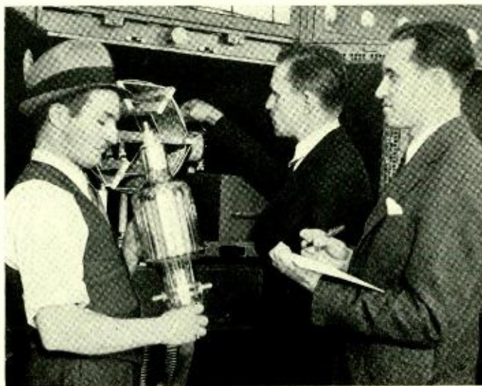
Inspecting the recently installed Western Electric 5000-watt transmitter for Station WTCN of the St. Paul "Pioneer Press" and "Minneapolis Tribune." Left to right, A. L. Lennon, Chief Engineer of the station, F. H. McIntosh, Bell Telephone Laboratories and J. M. Sherman, Federal Communications Commission
