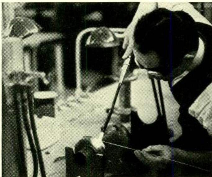
Brazing the water-cooled anode of a vacuum tube
