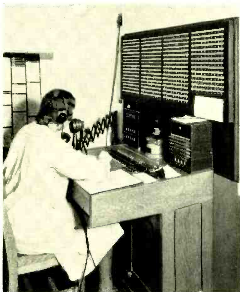
Paging position at the information center of the New York Hospital. The loud speaker control cabinet is at the left. Keys on the shelf connect the operator to the telephone system
