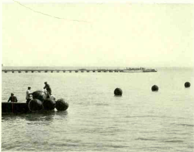
Marking buoys used in laying the Key West-Havana cable were balloons retained within networks of rope
