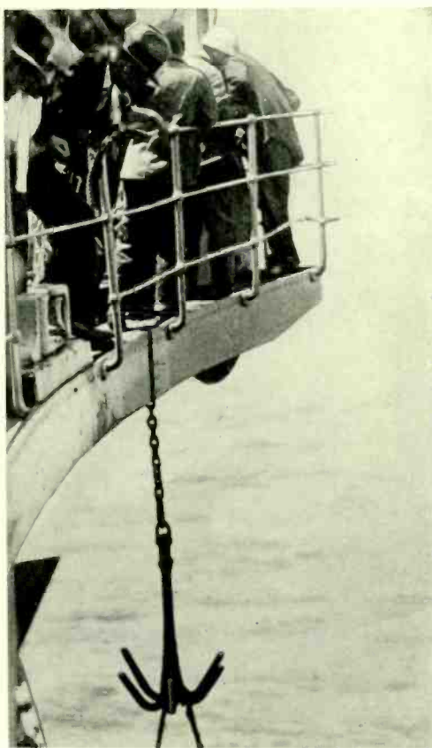
Fig. 4—A cable, damaged after it has been laid, is hauled aboard ship by a grappling hook and repaired
