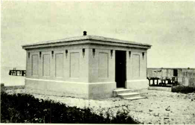
Fig. 5 — The cable hut at Key West
