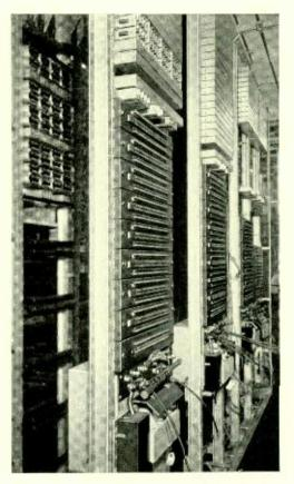
Fig. 5—A partially completed installation of relay-rack equipment to be associated with busy lamp signals
