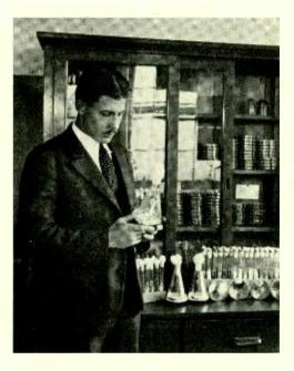
Our Timber Products laboratory has among its equipment pure cultures of eleven fungi which cause decay of wood. These microscopic plants are used to study various preservatives for telephone poles
