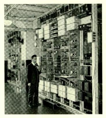
Fig. 3—F. A. Muccio at one terminal of a Type-C carriertelephone system
