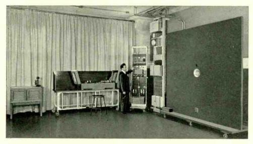
Fig. 5—Walls of the program observing room have been treated with rock wool to obtain a desirable reverberation time which may be varied by adjusting monk's cloth curtains at one end. In the background is a phonograph-reproducing set and on the right is a high quality loud speaker with baffle board
