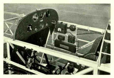
Western Electric radio-telephone equipment for itinerant flyers installed in Fairchild airplane
