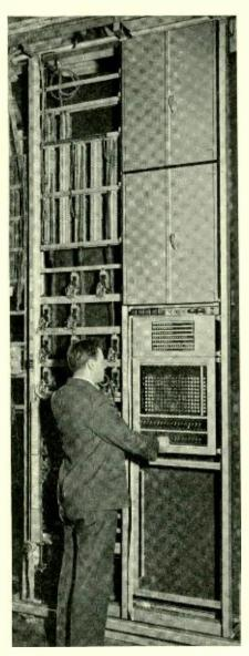
A standard test circuit for subscriber's senders in the systems laboratory
