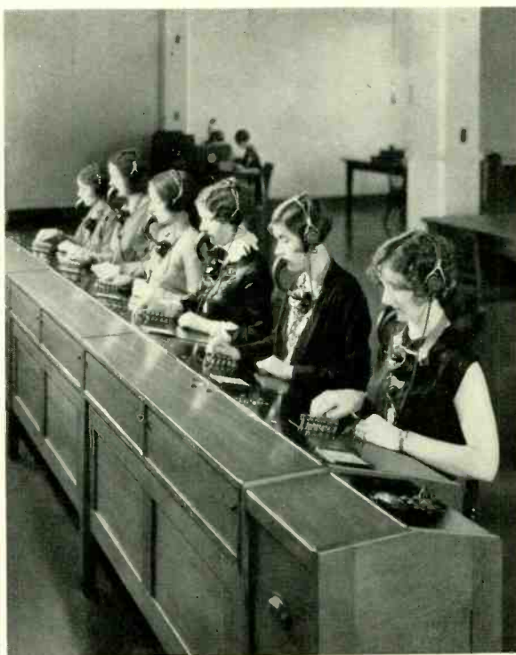
Fig. 2—Three sections of call-distributing "B" board
