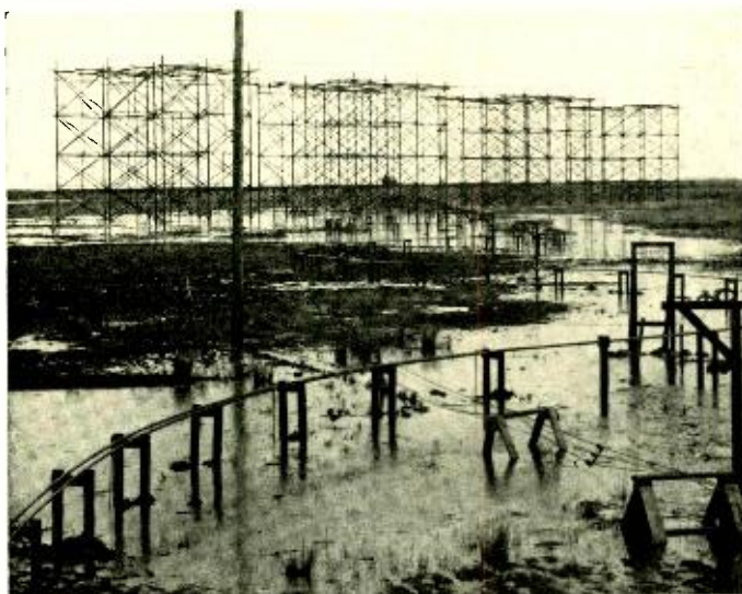
A receiving-antenna structure of the ship-to-shore radio system, at Forked River
