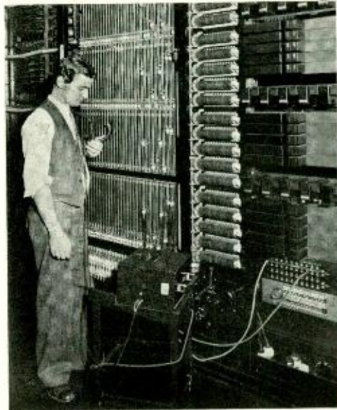
Fig. 3—Smaller than the “tea-wagons” are the box-type test sets, one of which is shown here in use at a B-position incoming-selector frame
