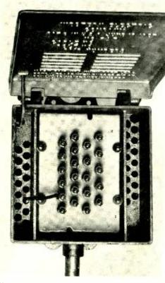
Fig. 4-No. 14 type cable terminal with porcelain block in place
